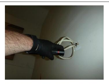
Loose hanging light fixture observed, suggest repairing for safety.
