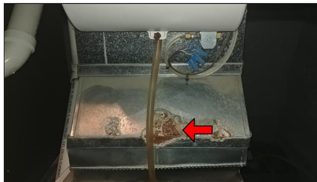
11.7 Item 2(Picture) Corrosion associated with leak from humidifier
