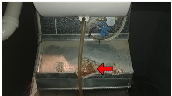
11.7 Item 2(Picture) Corrosion associated with leak from humidifier
