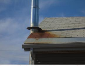
Curling shingles observed. Recommend review by a licensed roofer for repair or replacement, as necessary, prior to close.
