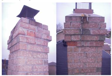
Flaking or spalling bricks noted. Suggest monitoring and repairs or rebuilding by a qualified chimney contractor when required.
