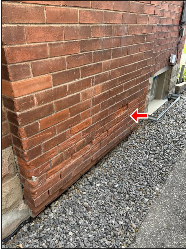
1.2 Item 1(Picture) spalling brick
