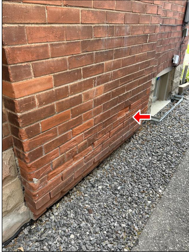
1.2 Item 1(Picture) spalling brick
