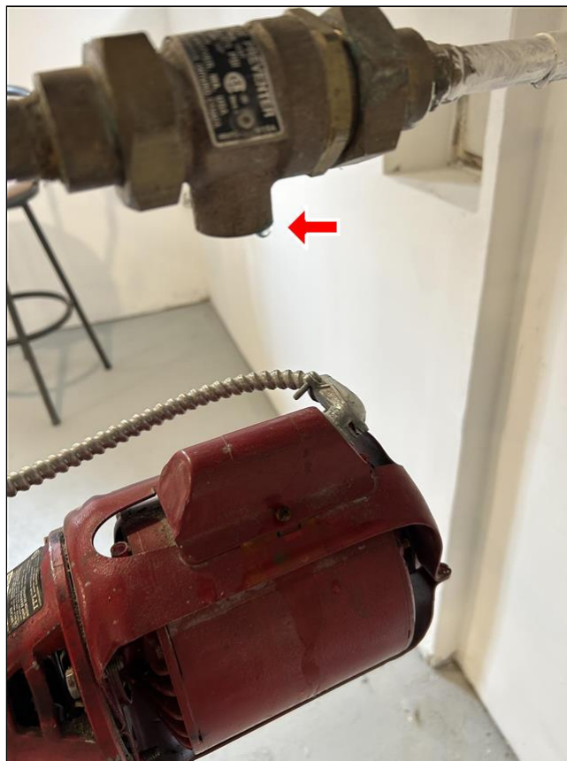
7.5 Item 3(Picture) leaking valve
