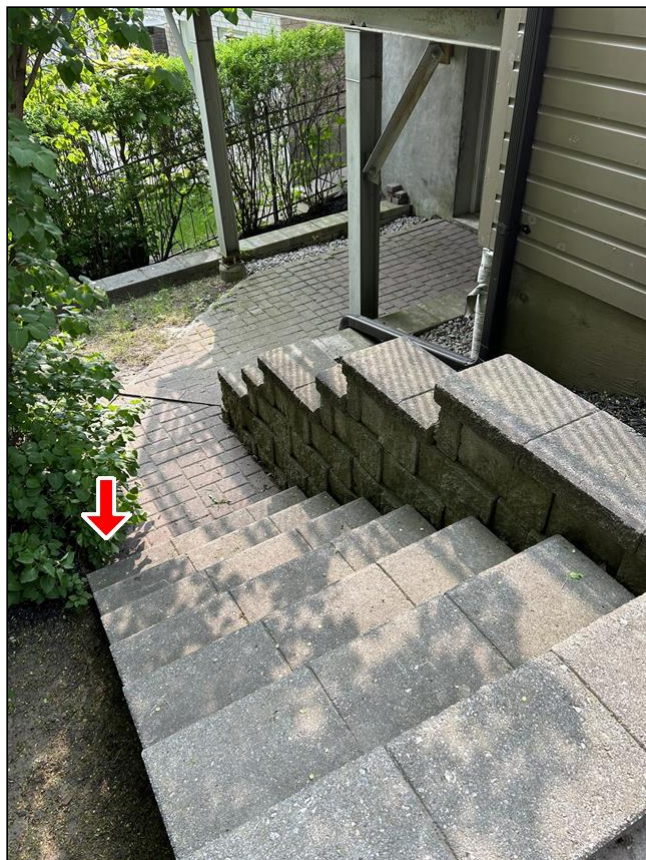
1.11 Item 1(Picture) missing railing
