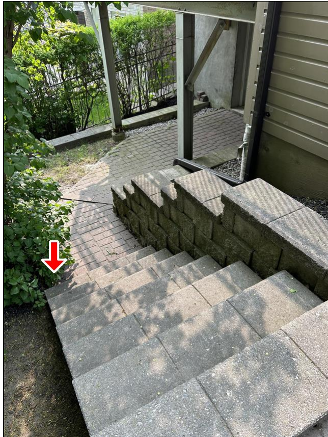
1.11 Item 1(Picture) missing railing
