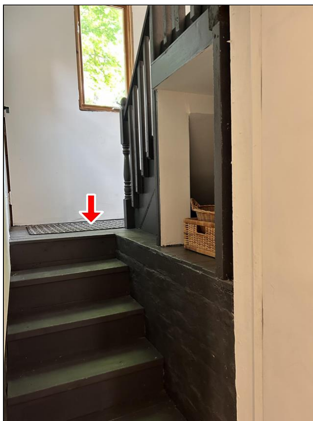
13.9 Item 1(Picture) missing railing
