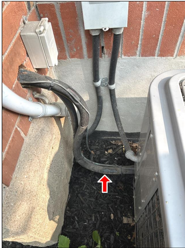
8.0 Item 2(Picture) deteriorated insulation
