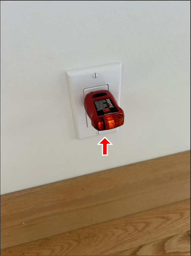
13.7 Item 2(Picture) reverse polarity
