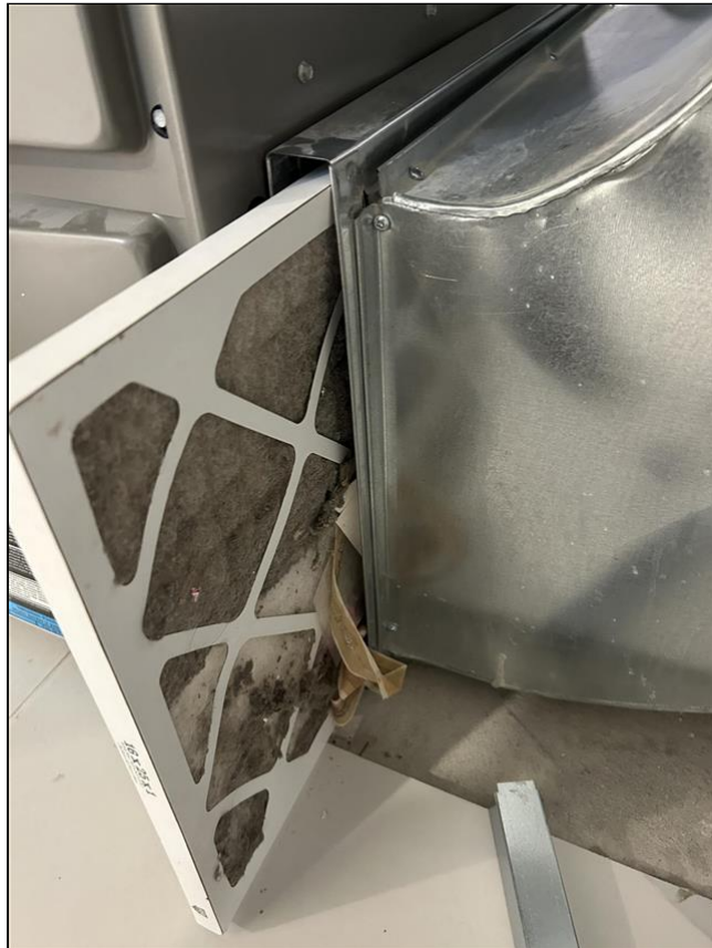
7.4 Item 1(Picture) filter condition
