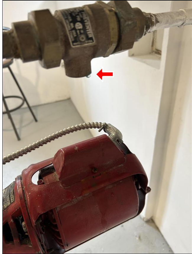
7.5 Item 3(Picture) leaking valve
