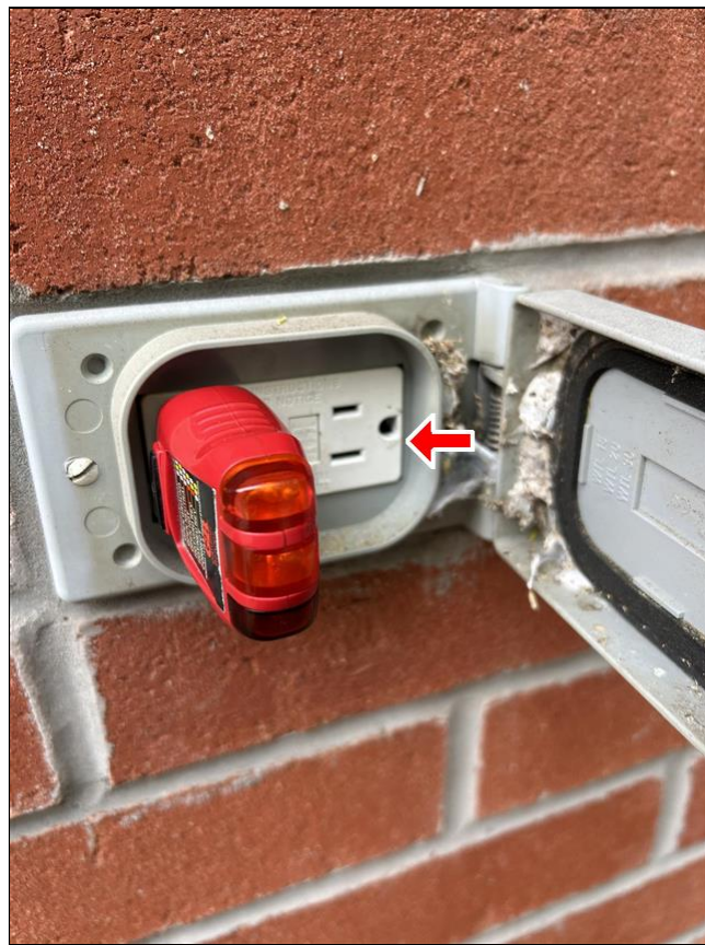
1.7 Item 2(Picture) defective GFCI
