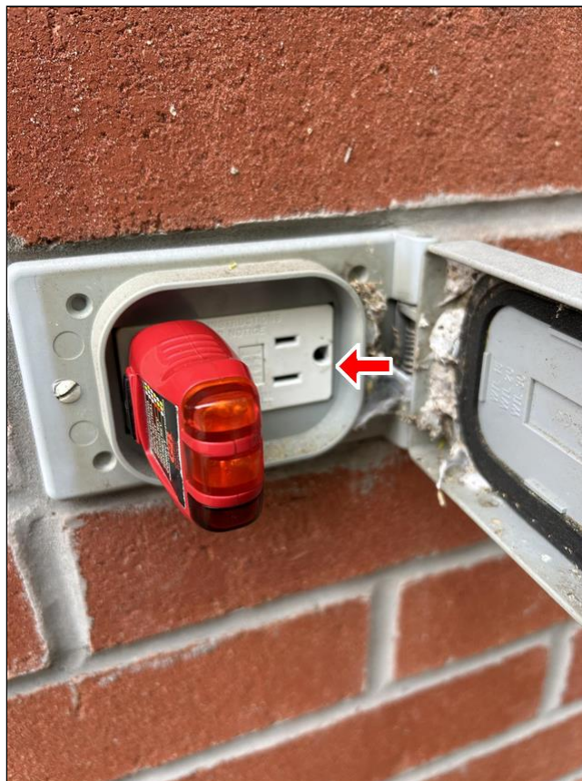
1.7 Item 2(Picture) defective GFCI
