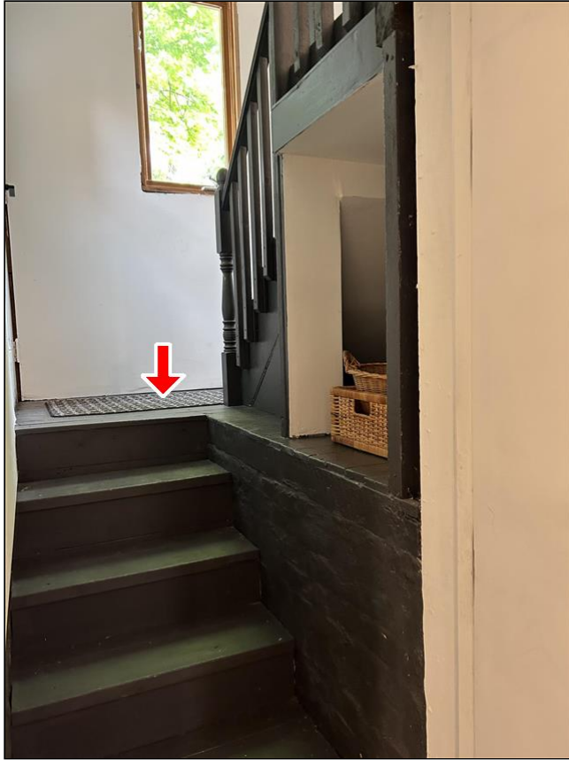
13.9 Item 1(Picture) missing railing
