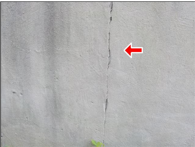
A. Item 1(Picture) Vertical crack
