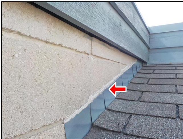
E. Item 4(Picture) Step flashing
