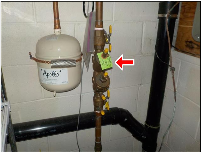
A. Item 1(Picture) Cross connection control
