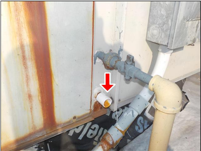
D. Item 2(Picture) Missing condensate trap
