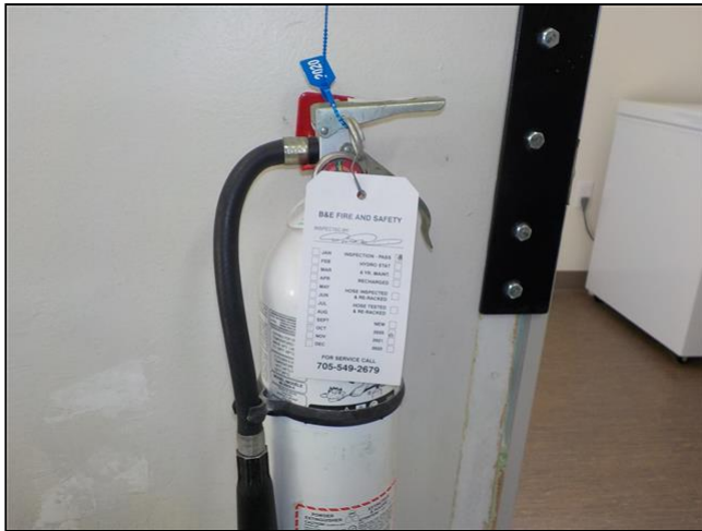
A. Item 3(Picture) Fire extinguisher inspection tag
