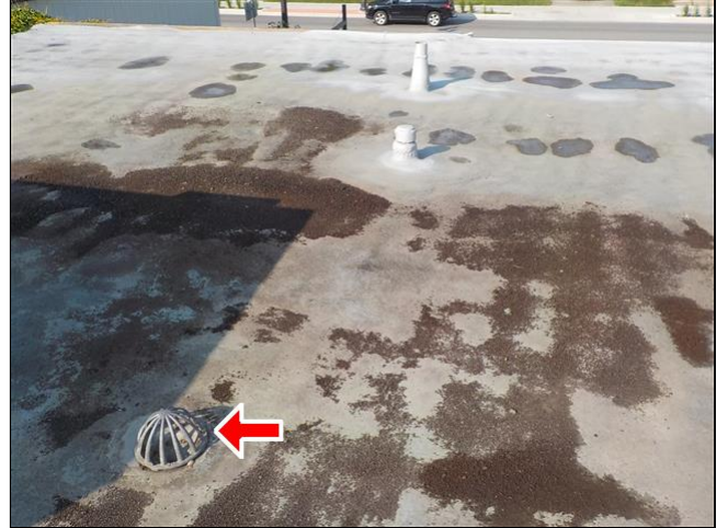
E. Item 2(Picture) Interior roof drain
