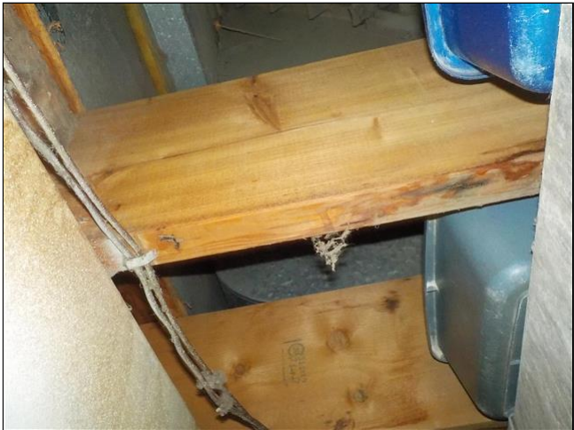
A. Item 2(Picture) Previous seepage below rooftop unit
