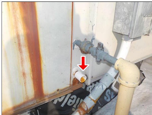
D. Item 2(Picture) Missing condensate trap
