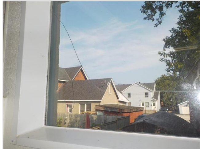
D. Item 2(Picture) Cracked window pane
