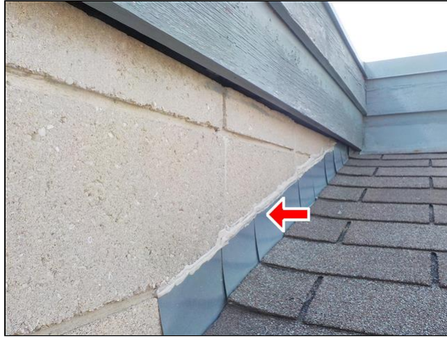
E. Item 4(Picture) Step flashing
