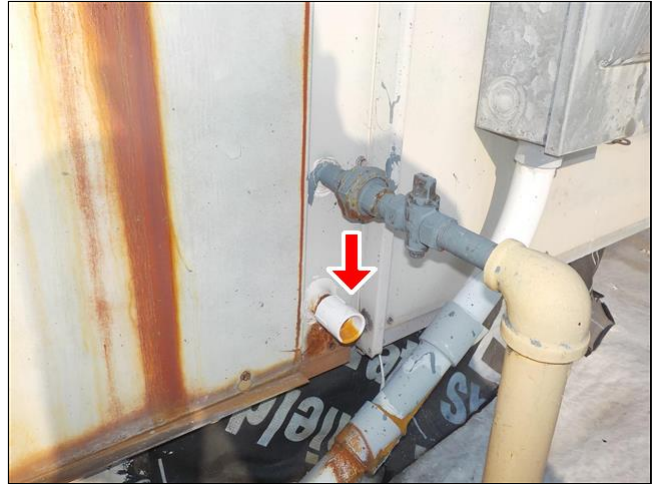
D. Item 2(Picture) Missing condensate trap
