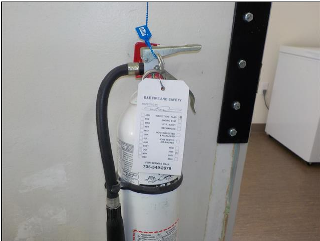
A. Item 3(Picture) Fire extinguisher inspection tag
