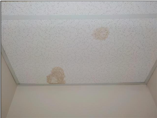
A. Item 1(Picture) Staining from previous seepage
