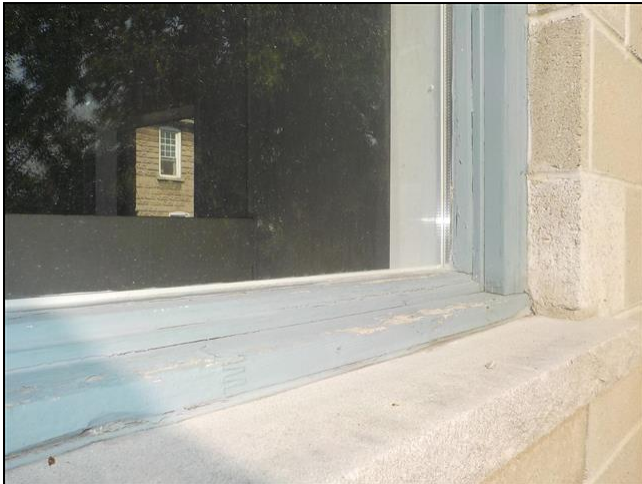
D. Item 1(Picture) Wood frame conditions
