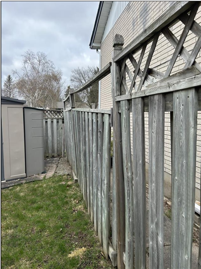
1.6 Item 1(Picture) fence conditions
