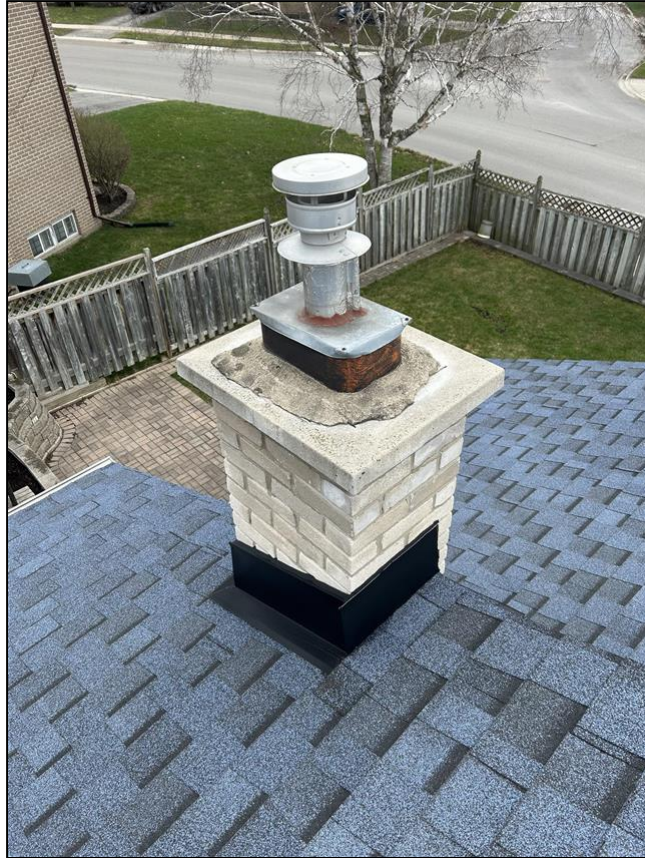
4.0 Item 1(Picture) chimney conditions
