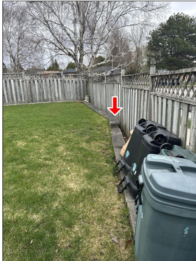
1.14 Item 1(Picture) retaining wall condition
