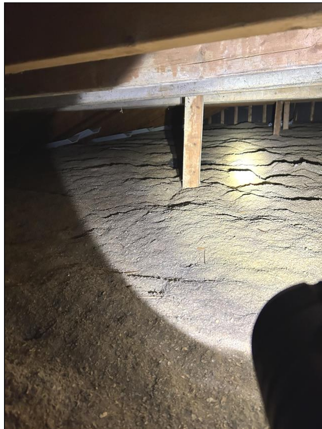
15.3 Item 1(Picture) insulation conditions
