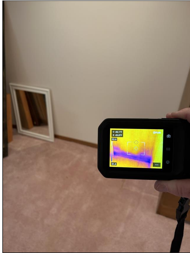
14.10 Item 1(Picture) thermal imaging
