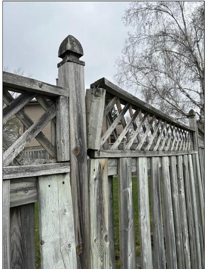
1.6 Item 2(Picture) fence conditions
