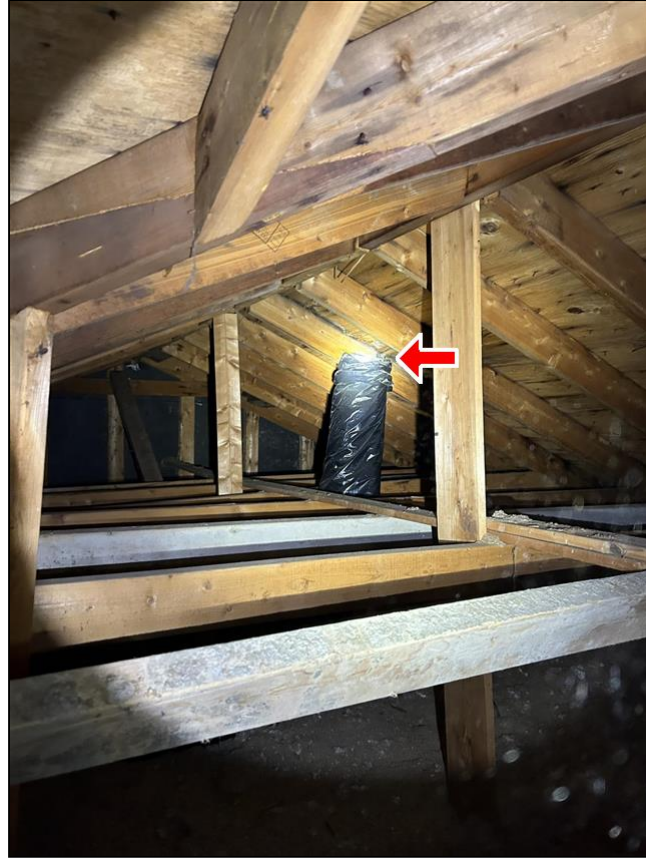
15.5 Item 1(Picture) bathroom vent
