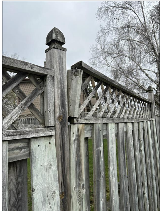
1.6 Item 2(Picture) fence conditions
