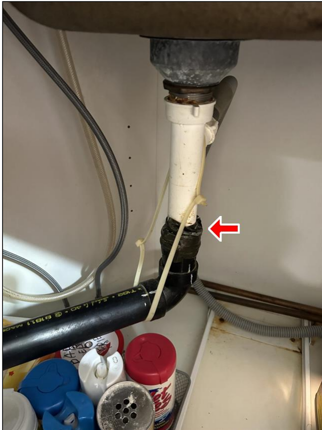
11.8 Item 1(Picture) drain repair
