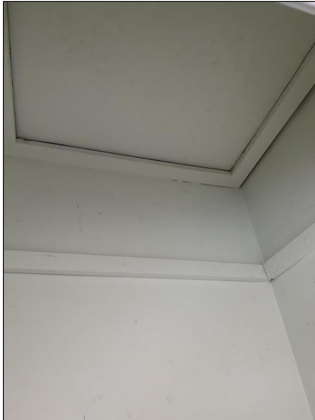
15.0 Item 1(Picture) attic hatch
