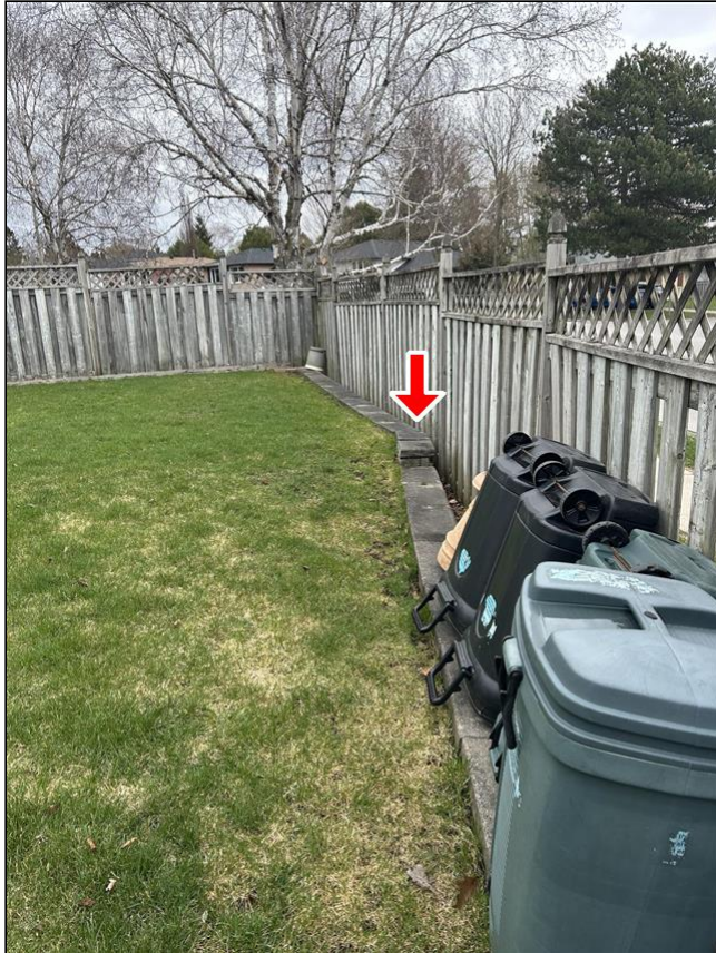
1.14 Item 1(Picture) retaining wall condition
