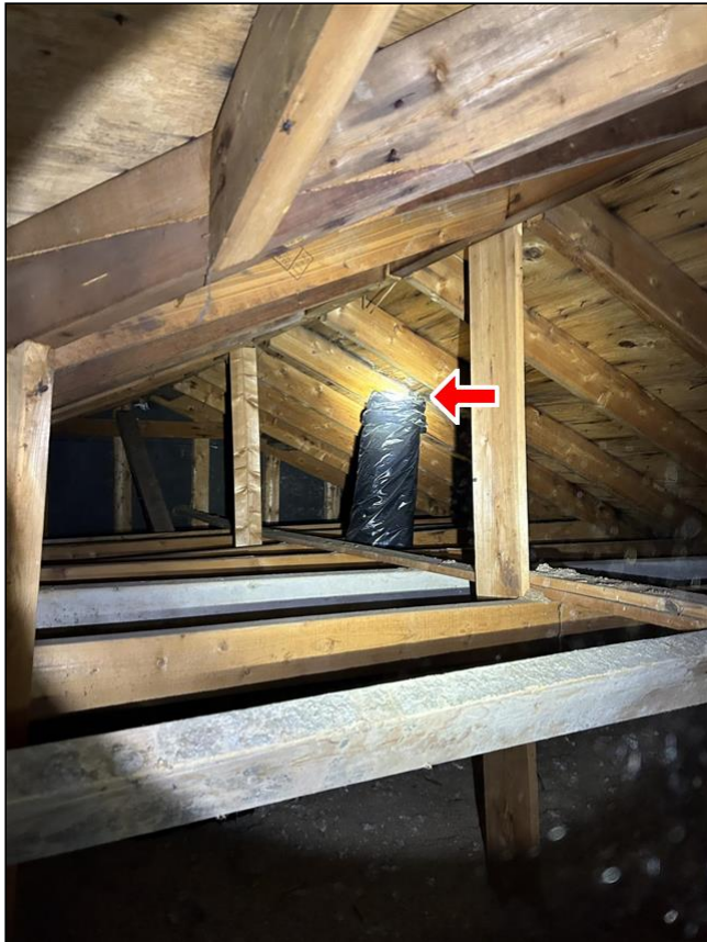
15.5 Item 1(Picture) bathroom vent
