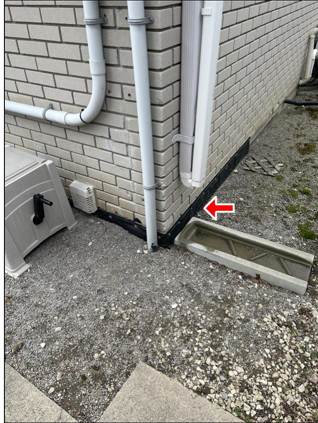
5.1 Item 1(Picture) waterproofing
