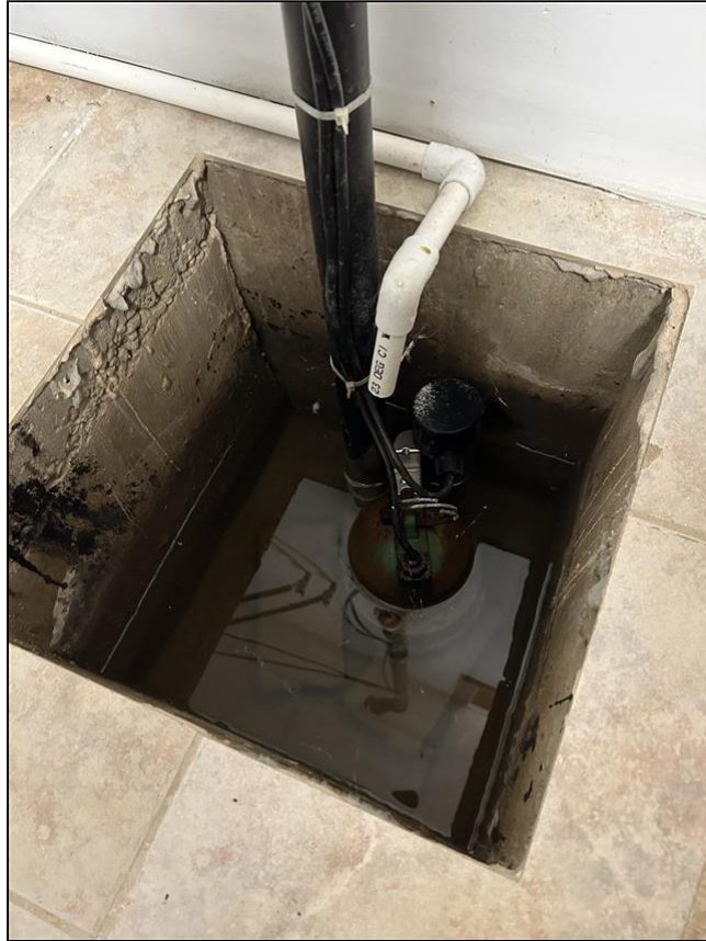
6.4 Item 1(Picture) sump
