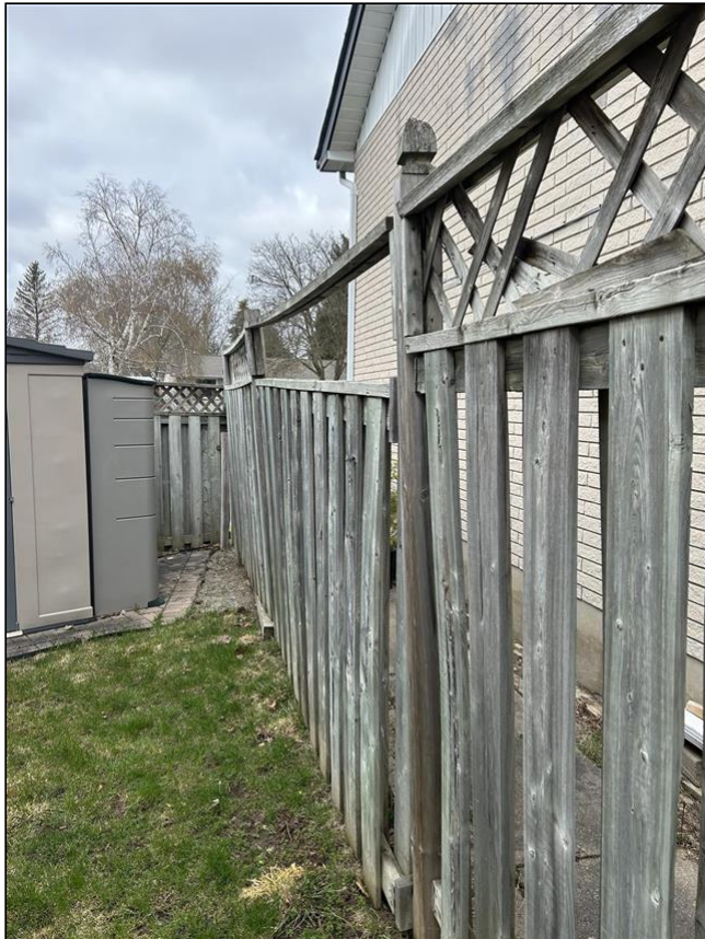
1.6 Item 1(Picture) fence conditions
