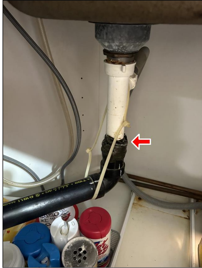
11.8 Item 1(Picture) drain repair
