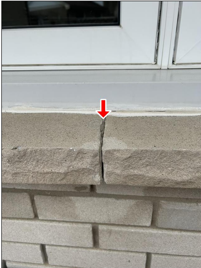
1.4 Item 1(Picture) sill joint
