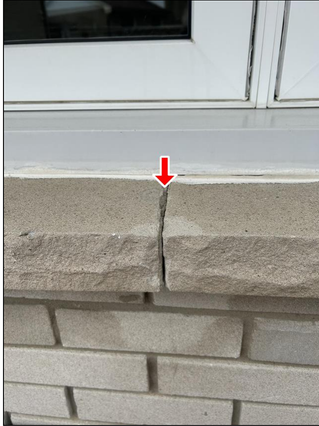
1.4 Item 1(Picture) sill joint
