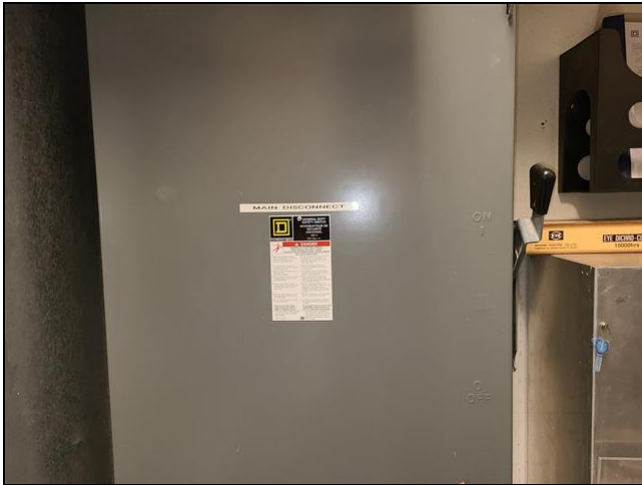
Main Electrical Shut Off
